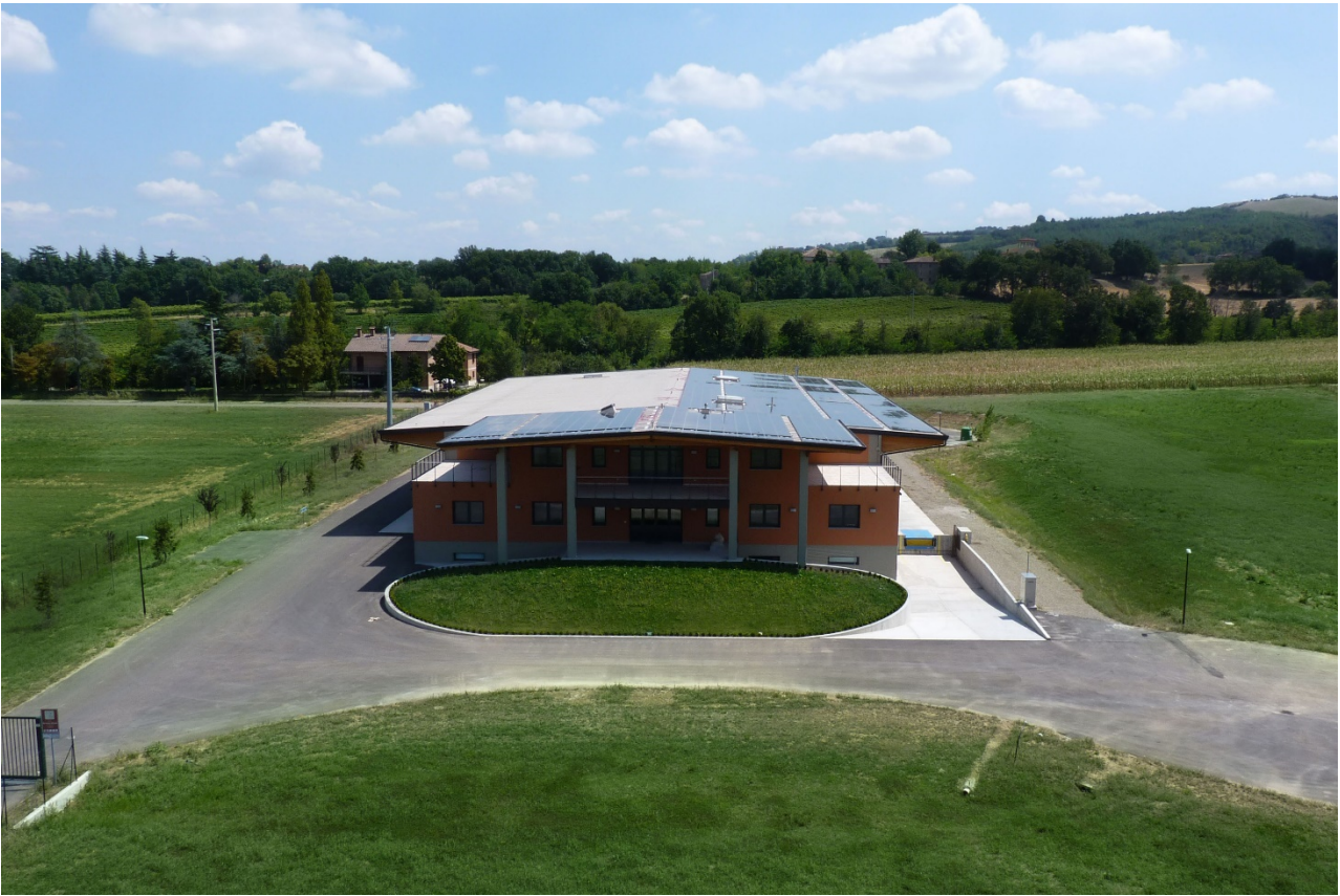
Aerial view from drone (solar cells on the roof)
